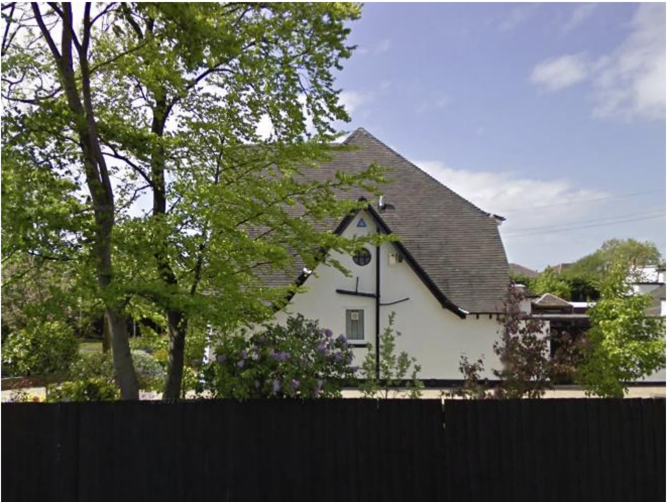
Figure 6: First-Floor Side Window non-Stained in 2009 (Source: Google Maps)
